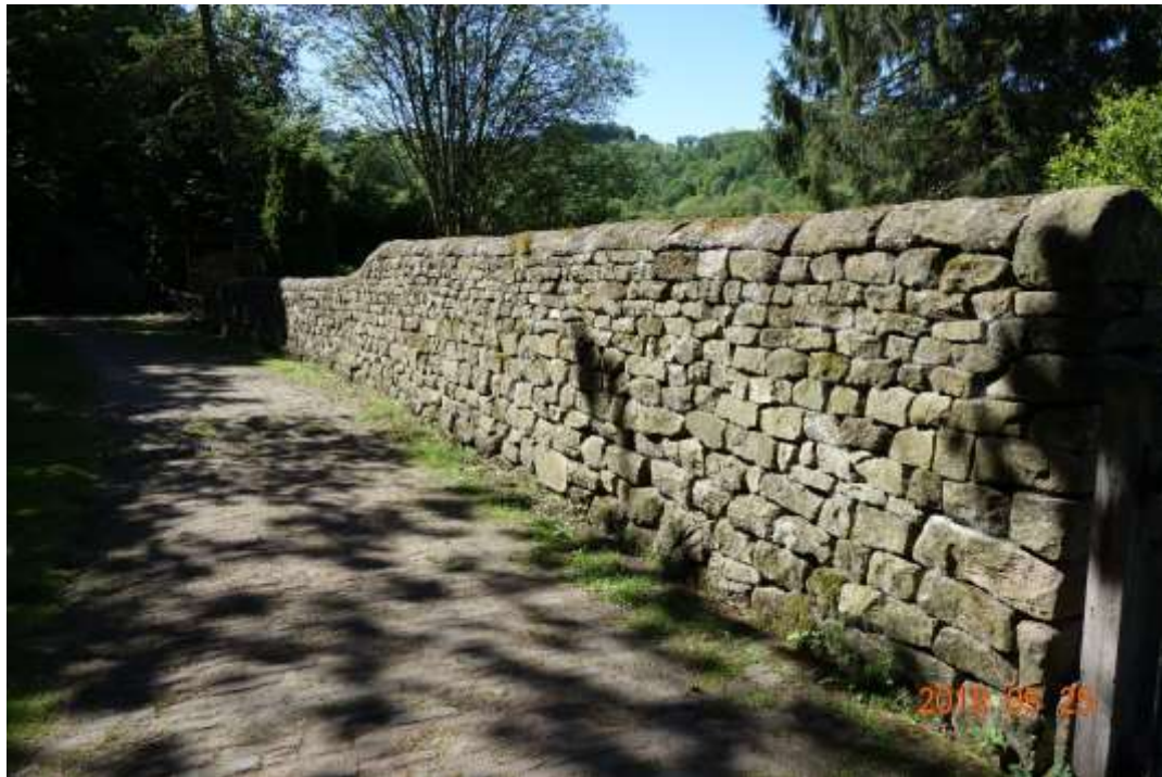
Dry stone wall at Lea Wood
